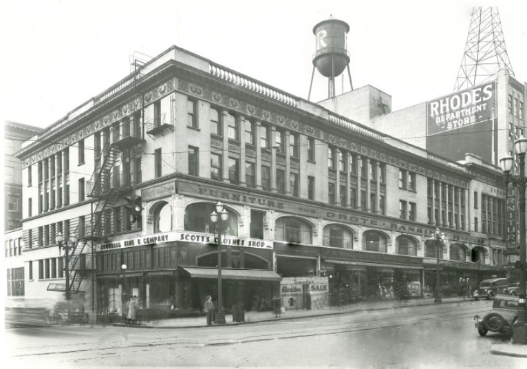
55. Arcade building, Seattle, 1932.
